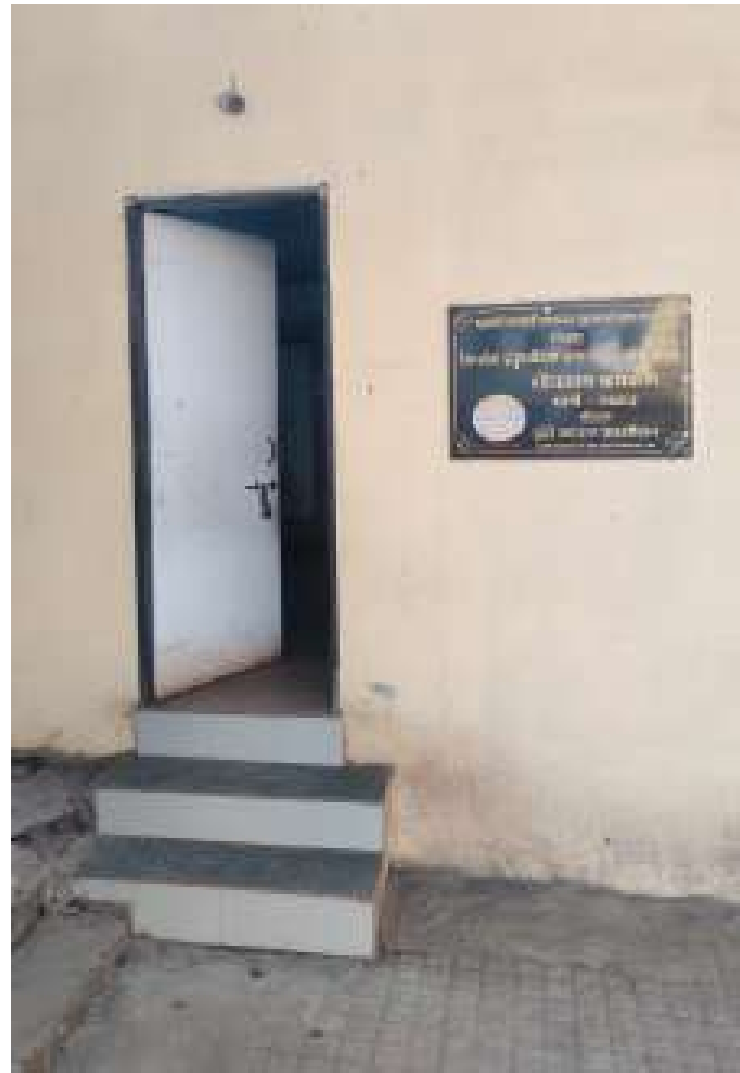
NEW CONSTRUCTED TOILET BLOCK IN SCHOOL
